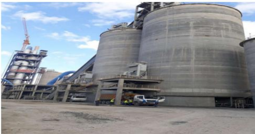
Figure I.12: Silos stockage de clinker.
