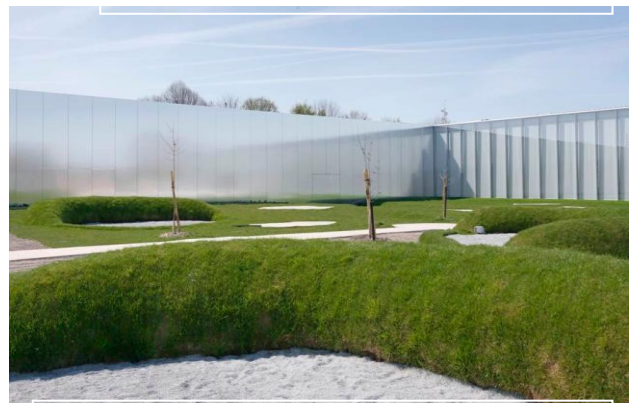
Figure 126: l'utilisations du verre a façades Source : https://www.inexhibit.com/mymuseum/louvre-lens/
