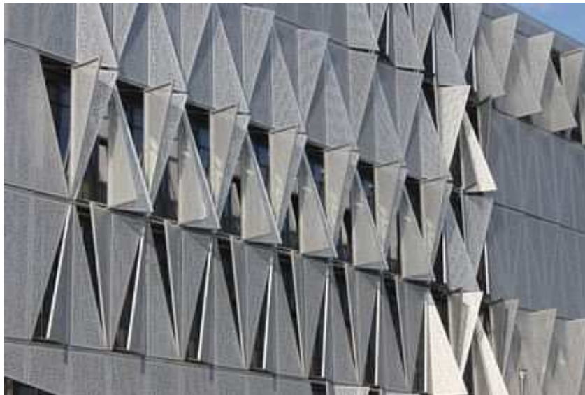
Figure 2.13: Adaptive building's skin responding to solar radiation
