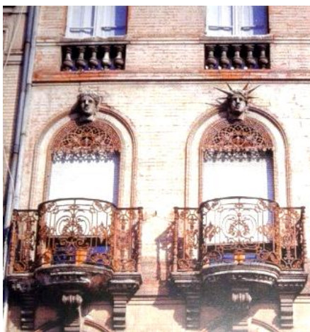
Figure I-32 : Balcon. Source : GAUTHIEZ, 2003.
