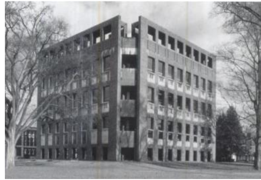
Figure I-21 : Articulation négative, joint creux Louis Kahn, librairie, Phillips Exeter Academy, Exeter, New Hampshire, 1965-72. Source : VON MEISS, 1986.
