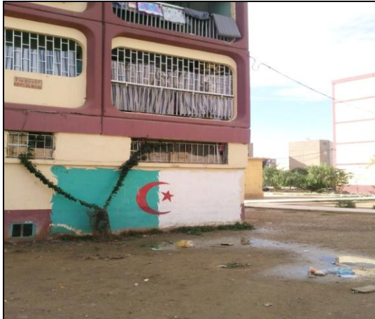
Photo.62: Stagnation des eaux
