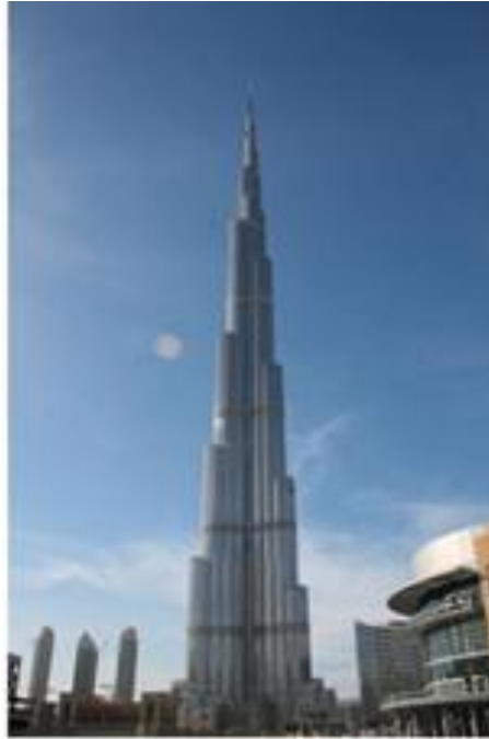
Figure A.3 Burj Khalifa building (Poulos 2016)
