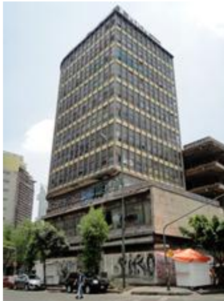
Figure A.1 La Azteca building, Mexico ( Poulos 2016)
