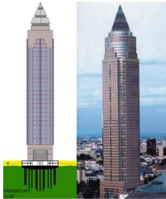
Figure A.9 Messeturm Tower of Frankfurt city, Germany (Katzenbach and Leppla 2015)
