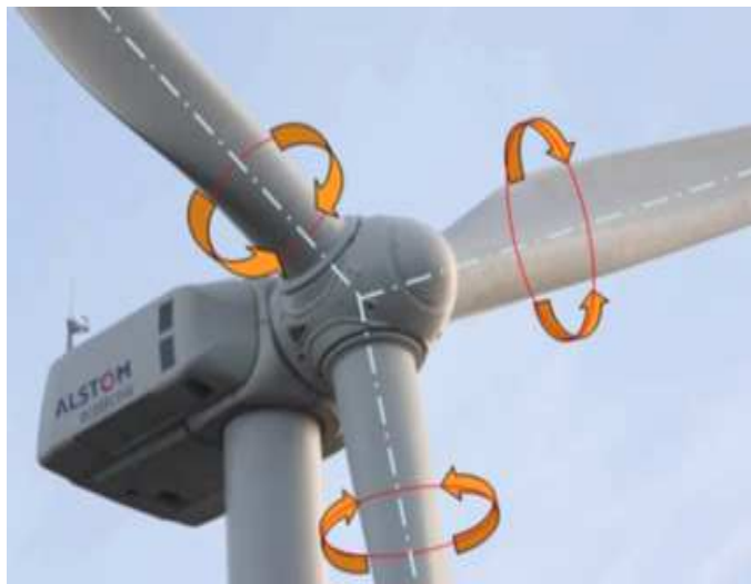
Figure II.6 : Orientation des pales.
