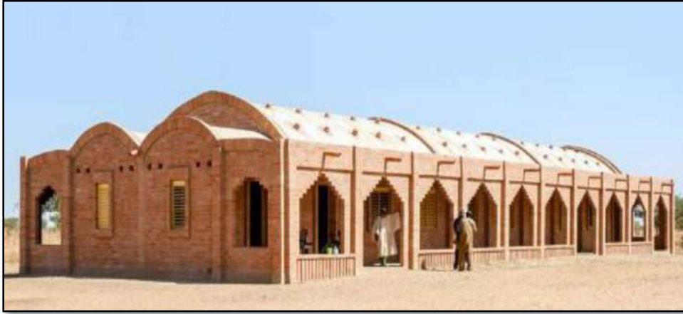
Figure 2. 5: An elementary school made of compressed earth blocks in Tanouan Ibi village.
