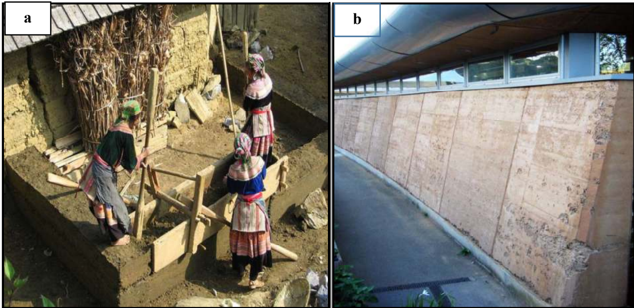
Figure 2. 2: a) Method of making an earthen rammed wall for a Hmong house in Vietnam ; b) The entrance edifice of the Eden Project in Cornwall, England, UK.
