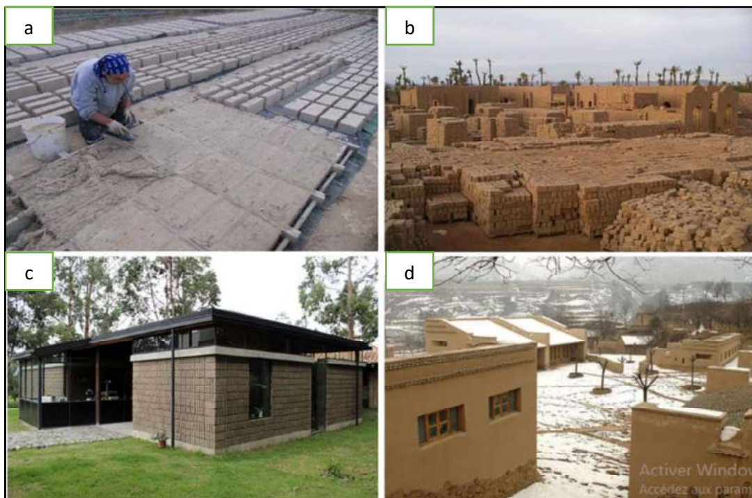
Figure 2. 4: a) Manufacture of adobe at small industrial scale in Palencia, Spain. b) Massive storage of adobes, Villa Janna, Marrakech, Morocco. c) Contemporary unplastered adobe house, Lienzo de barro, Ecuador. d) Contemporary adobe nursery school plastered with a fine soil render, Maosi, China.[49]
