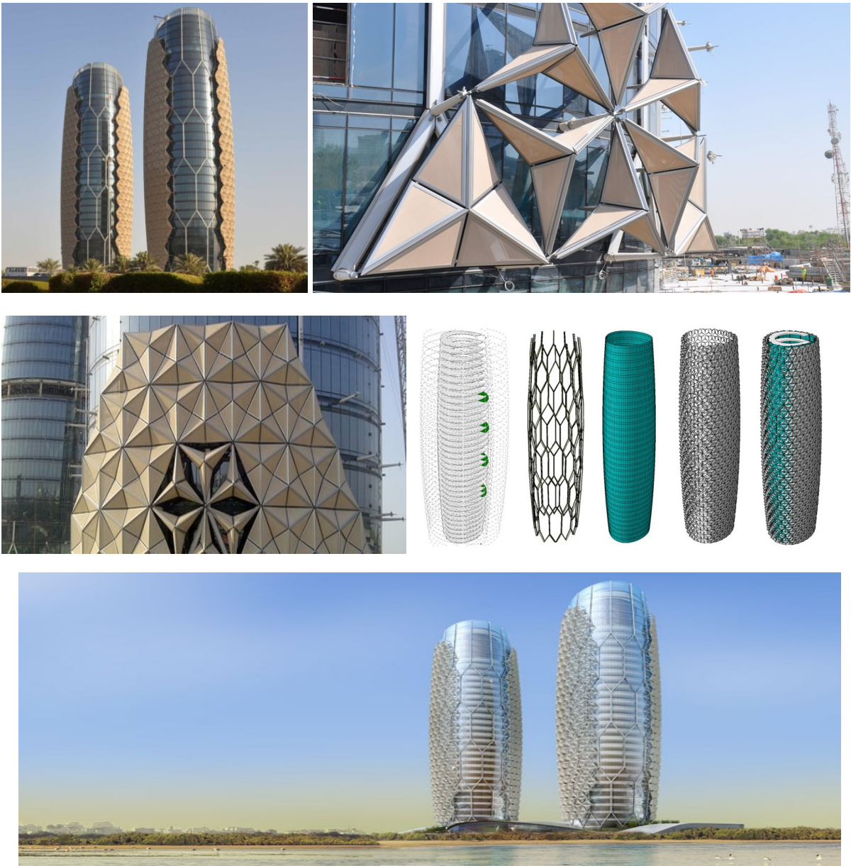
Figure 2.5: Al Bahar Towers in Abu Dhabi (Source: https://www.archdaily.com/270592/al-bahar-towers-responsive-facade-aedas )
