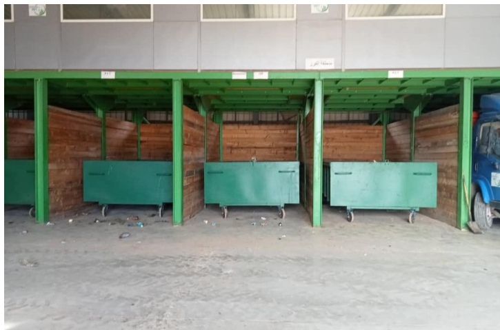
Figure 42: Material Collection Bunkers
