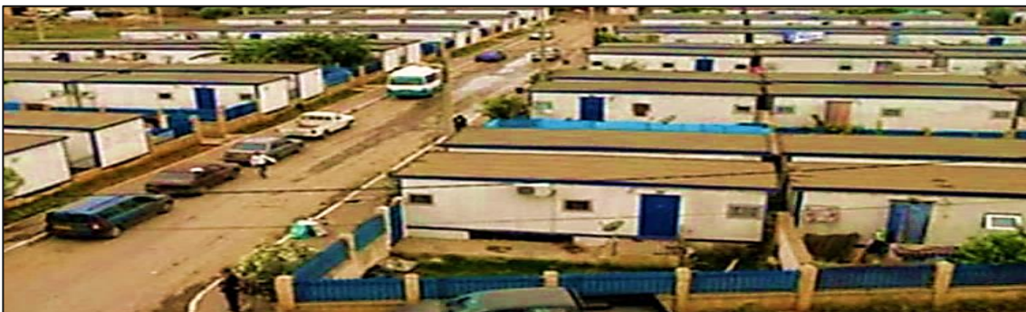
Figure 22: Prefabricated Dwellings of Chlef City
